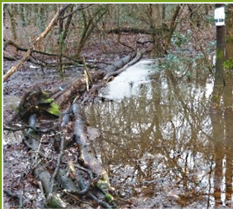
A leaky dam, providing attenuation in Park Wood (along Coppickers Channel) on 28th January 2021.
