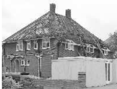
Demolition of the large family house at 41 Kingsend is already underway
