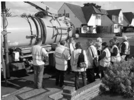
Gully cleaning in Eevelyn Avenue
